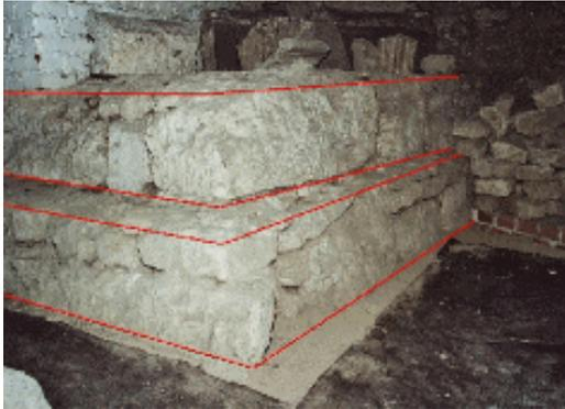
*Figure 5 Tacheometrically measured shape characteristics as a geometric base for the integration of manually drawn archaeological plans*
